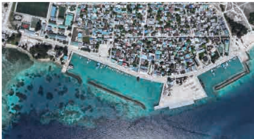
Aerial View of the Kelin Electric Clean Energy Supply Projects in the Maldives Archipelago
